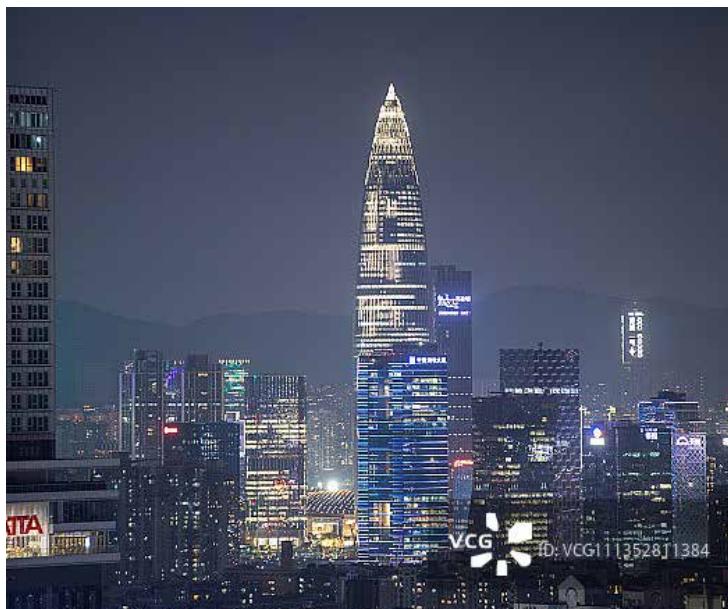
China Resources Shenzhen Bay Headquarters
